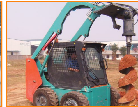
Construction in Changsha
